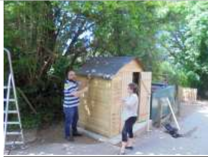
PTA Chairman Russ Stevens building the new shed.
